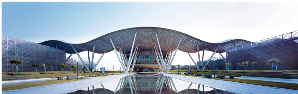
Qatar Science & Technology Park, Doha Year constructed: 2009 · Material: J57S
