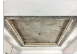
Photo No. 2 Receiver Room View of Test Specimen Installation
